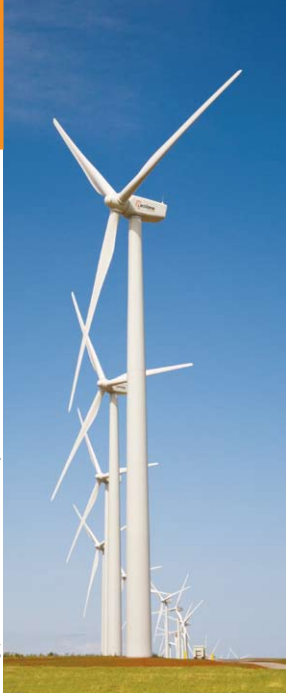
Photograph of ACCIONA's Red Hills Wind Farm courtesy of ACCIONA.
